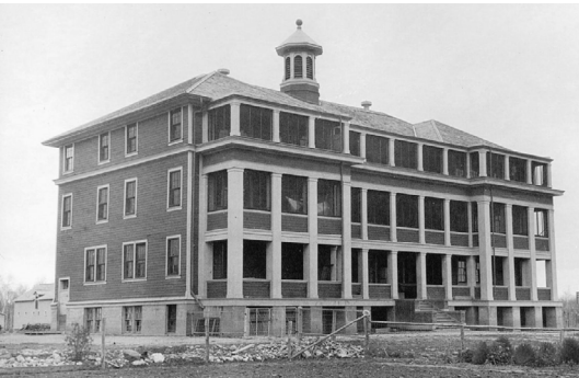
Figure A.31. Photograph showing the MacKay Indian Residential School (file P7538-954, Missionary Society of the Church of England in Canada Fonds, General Synod Archives, Anglican Church of Canada).
