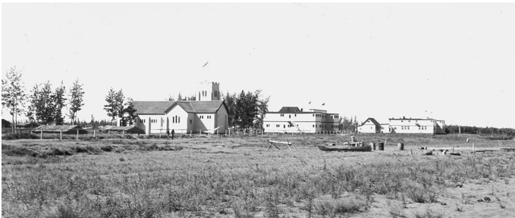
Figure A.59. All Saints Cathedral, Hospital and Residential School, Aklavik, Northwest Territories, n.d. (file P9314-137, Bessie Quirt Photograph Collection, General Synod Archives, Anglican Church of Canada).
