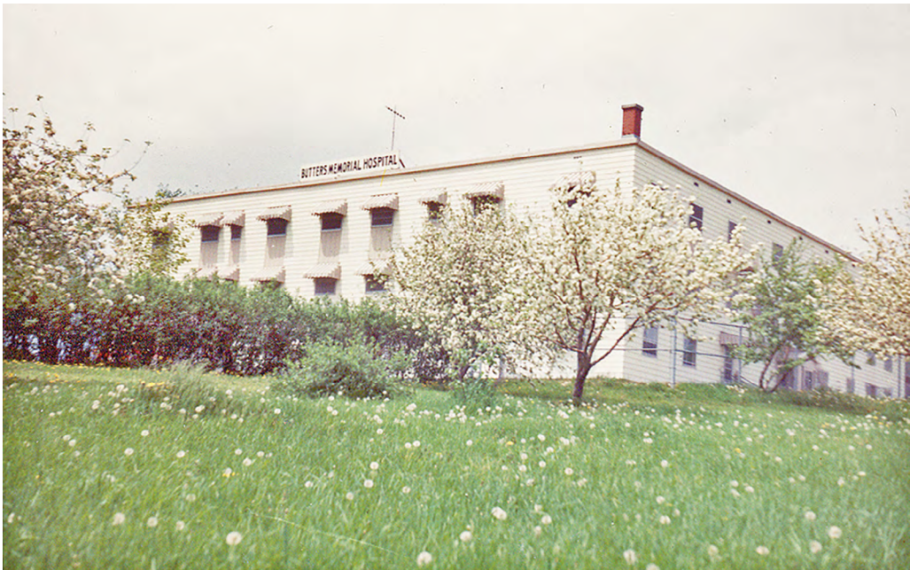
Figure 3.23. The Cecil Butters Memorial Hospital (from Butters Foundation).
