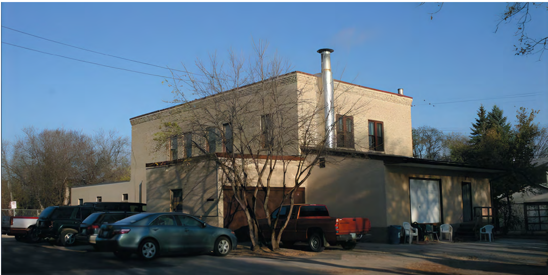
Figure 2.11. Photograph showing the powerhouse and laundry building in the Good Shepherd Marymount Complex (City of Winnipeg, Murray Peterson, Heritage Report: 442 Scotia Street, Marymount School Complex, December 2011, https://legacy.winnipeg.ca/ppd/Documents/Heritage/HeritageResourcesReports/Scotia-442-long.pdf ).
